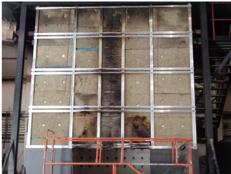
Photo No. 17 Exterior Cladding Removed (Post-Test)
