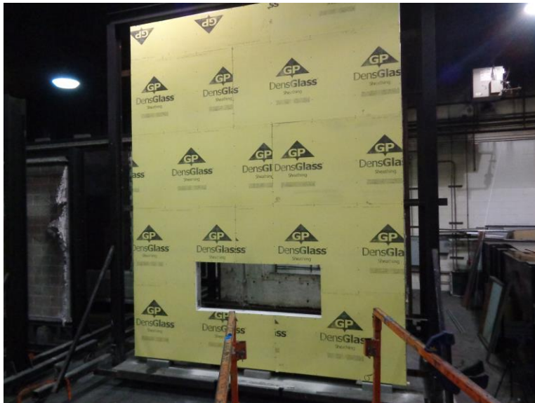
Photo No. 2 Exterior Sheathing Installed
