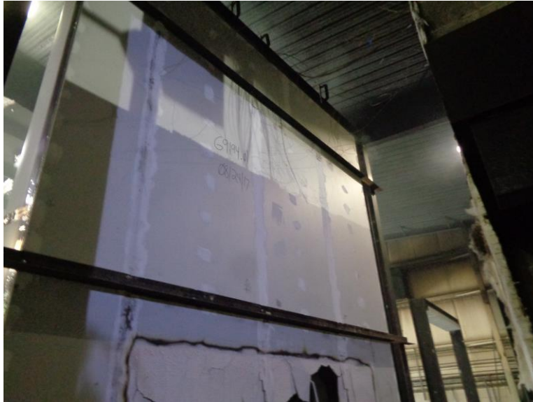
Photo No. 14 Second Floor Interior Gypsum (Post-Test)
