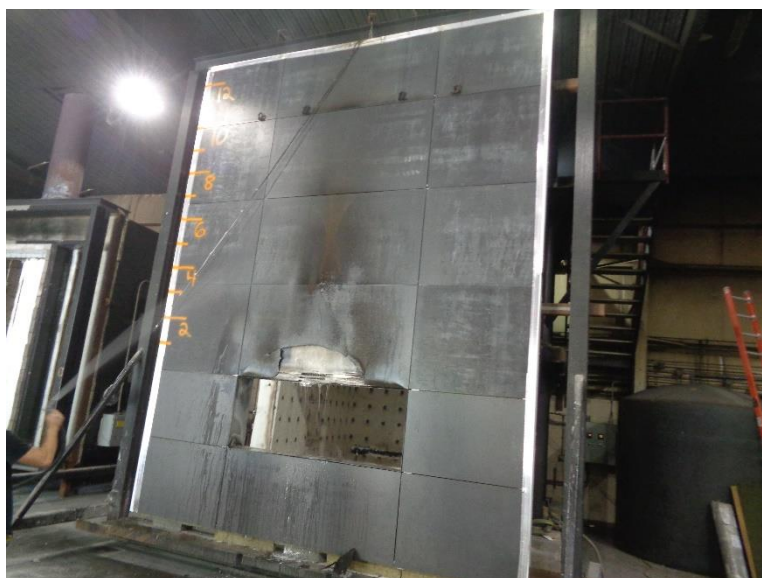
Photo No. 15 Exterior Surface (Post-Test)
