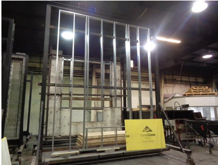
Photo No. 1 Completed Core Wall
