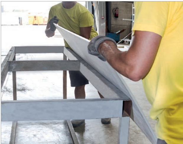
Image 9: Placing a Neolith Slab on a bench
