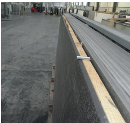
Image 3: Plank in the backside of the slab
