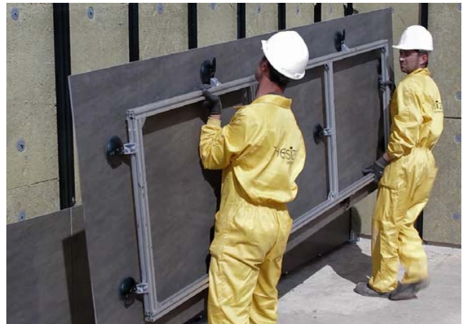
Image 7: Slab handling with Suction Frame
