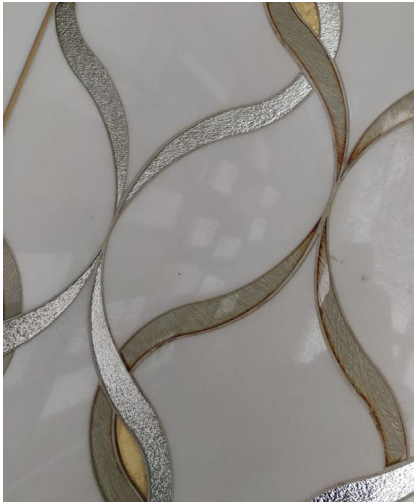
Fig 38 Example of contamination from iron
