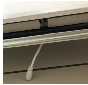
Fig 34 Example of slot for the electric wire
