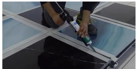
Fig 35 Sealing the gaps using neutral silicon
