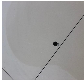
Fig 33 Example of hole for the electric wire
